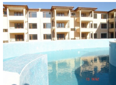
Kranevo Paradise Gardens 1, Kranevo
