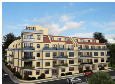
PLATINUM RESIDENCE III, Sofia
