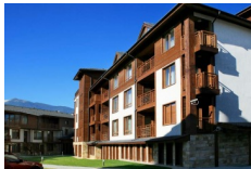
Adeona Residence, Bansko
